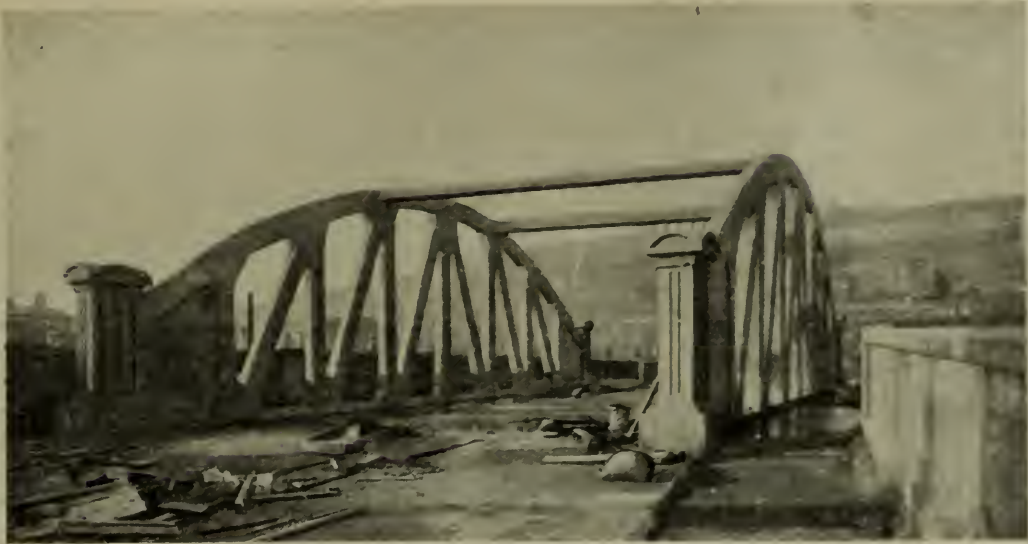
FIG. 2. DOVER AND DEAL RAILWAY BRIDGE.
